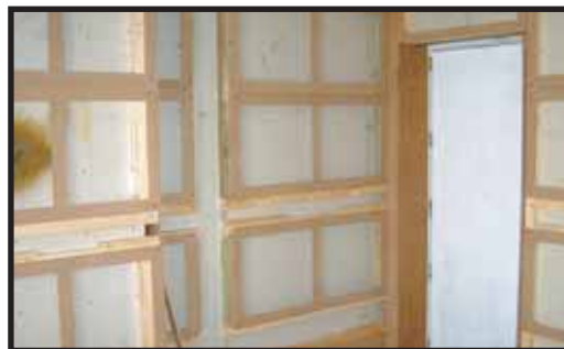
Frames awaiting material.
